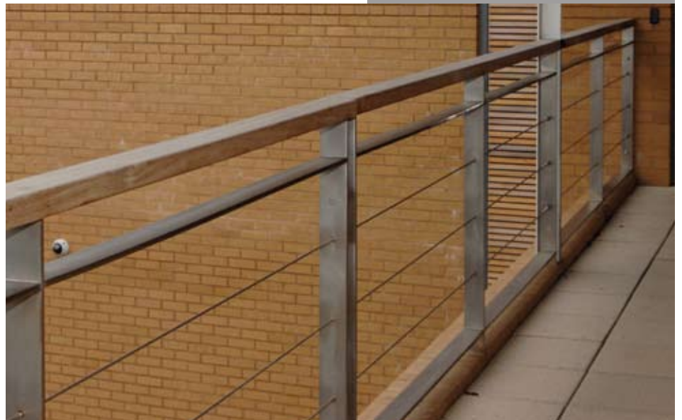
Ash handrails and radiused end detail.
