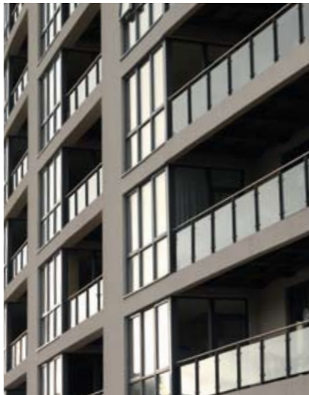
The installation was co-ordinated to accommodate the contracts phased completion.
