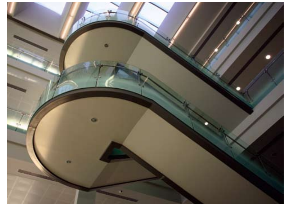
Curved and laminated glass with fritted screen printed pattern.
