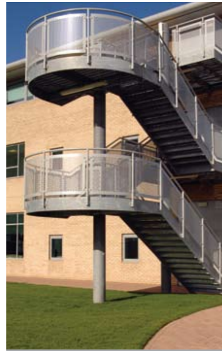
External feature fire escape with central column supports, curved landings and perforated infill panels.
