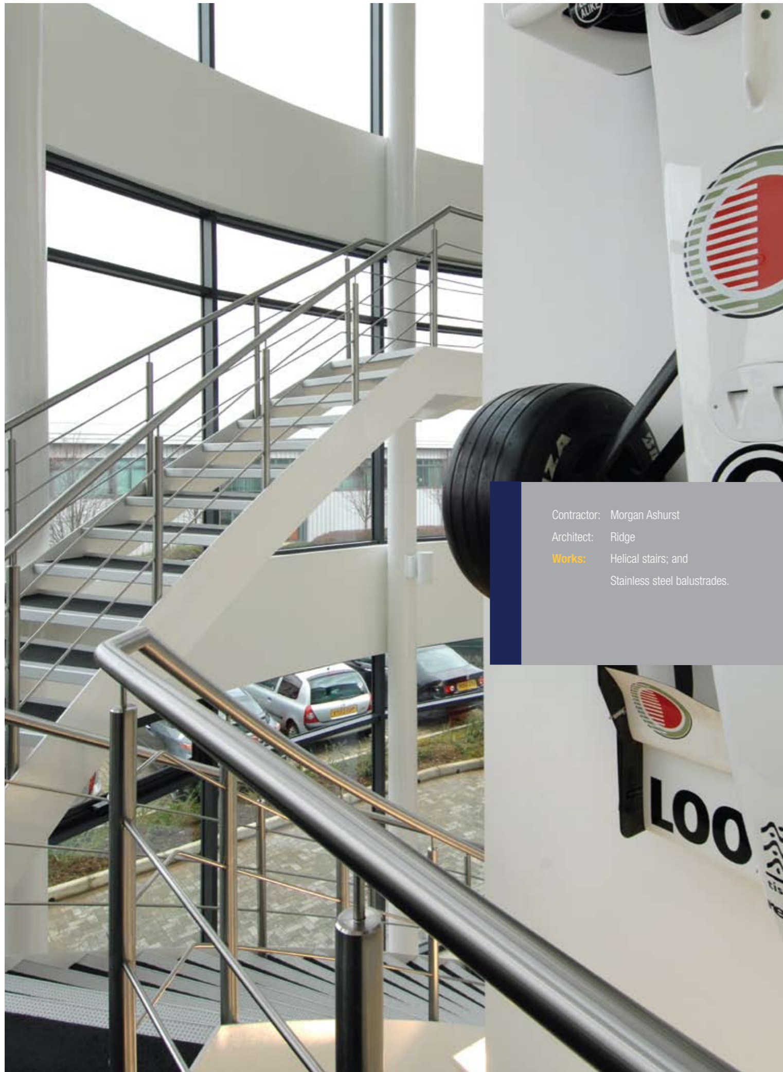
The main structure was supplied powder coated, thus providing a fully finished product, which required no further work by the main contractor.
