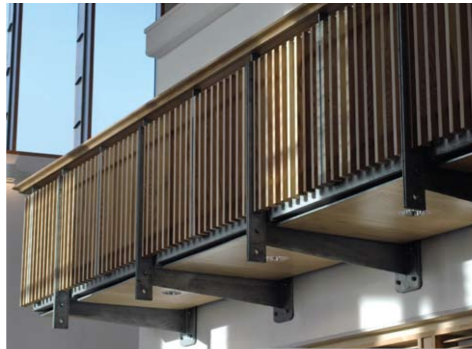
Cantilevered gallow brackets support the walkways over two storeys.
