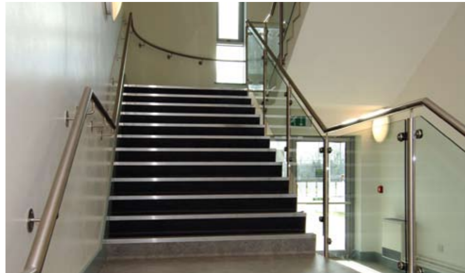
Internal balustrade is fitted as the project nears completion.
