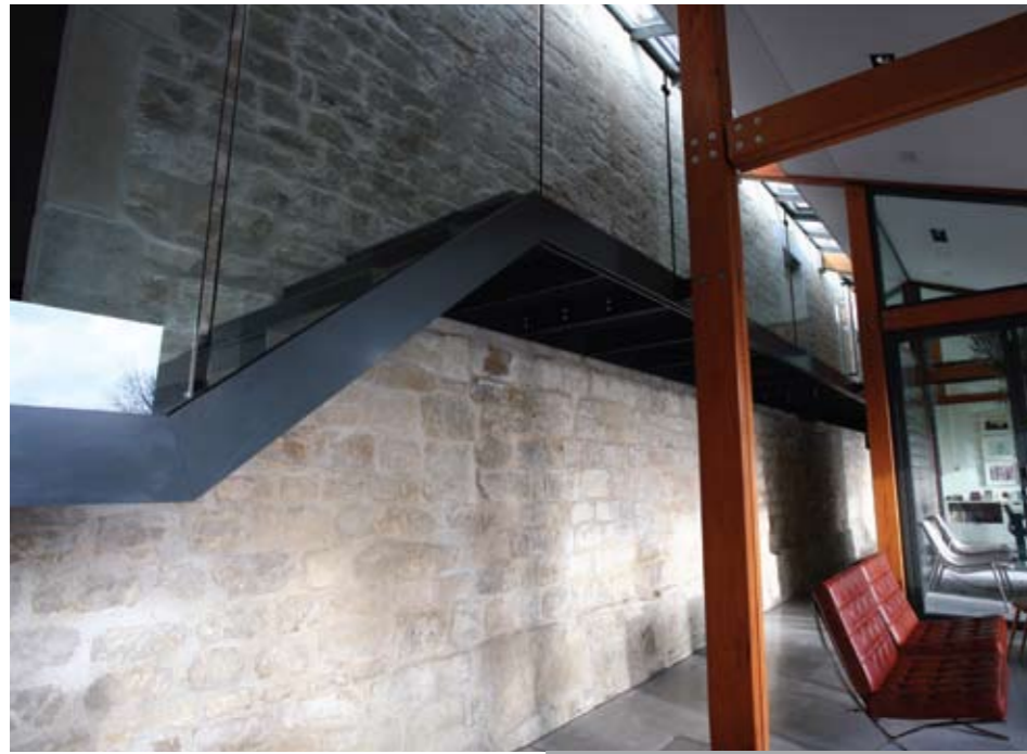
The very shallow stringer detail and appearance of the structure being self-supporting was an important design brief.
