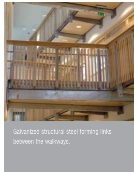
Galvanized structural steel forming links between the walkways.
