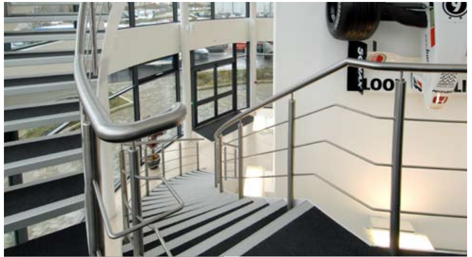
Horizontal and raking bar infill balusters and handrails, all in satin finished stainless steel.
