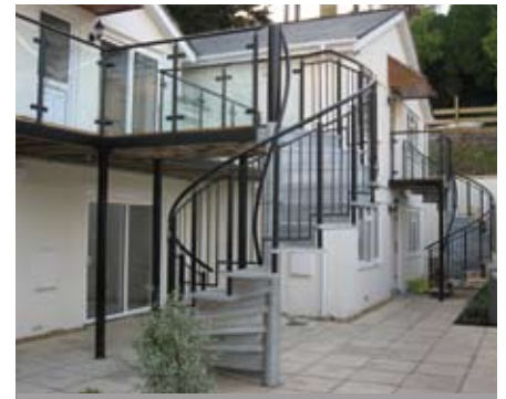
Residential galvanized stair with powder coat balustrade.
