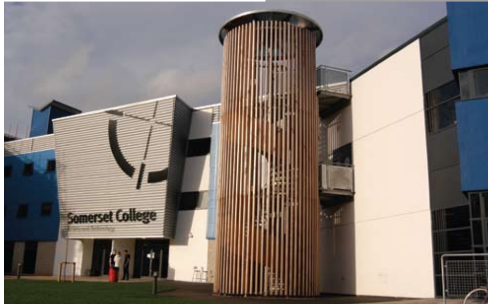
Powder coated stair and balustrade with s/s handrail.
