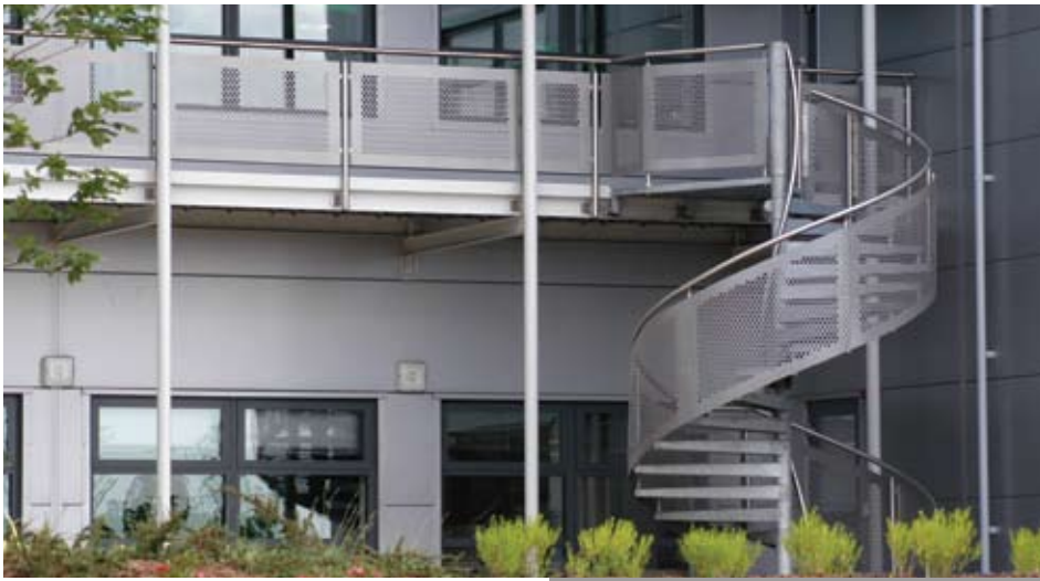
Galvanised stair with stainless steel handrails and terraced balustrade.
