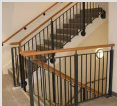
Bar infill powder coated balustrade with hardwood handrails. Southgate, Sir Robert McAlpine
