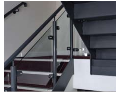
Mild steel powder coated structure and balustrade with glass infill panels.
