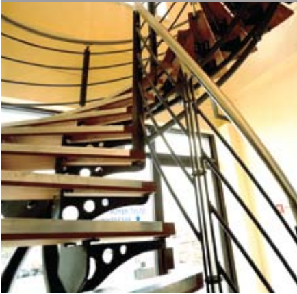
Powder coated cantilevered structure with timber treads and s/s wire infills.
