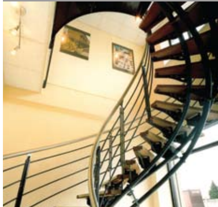
Flat string with timber treads and stainless steel handrails.
