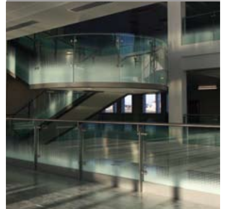
12mm clear laminated heat-soaked and toughened feature detail.
