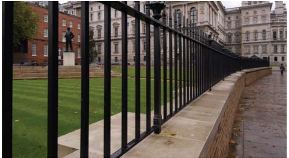
Heritage railings with cast finials.
