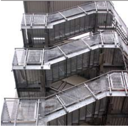
Galvanized structure and balustrade with mesh infill panels to balustrade.
