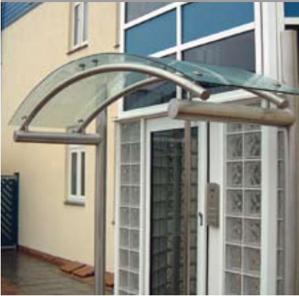
Galvanized structural steel, roof covering by main contractor.
