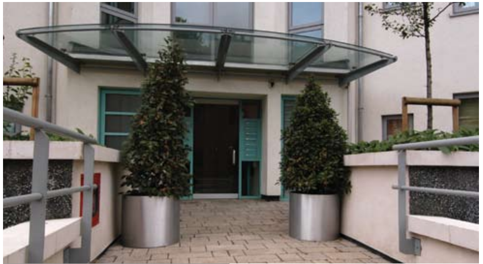
Zinc sprayed and powder coated structure with 15mm toughened and heat-soaked glass.
